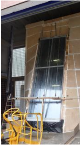
Figure 14: Water penetration test
