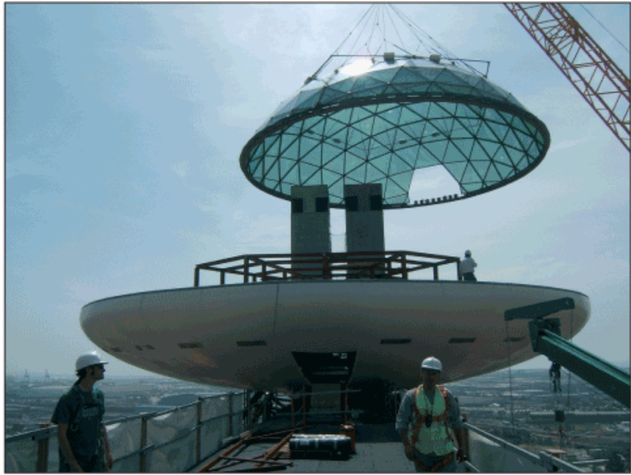
Fig. 4: Final positioning of the dome on top of the tower
