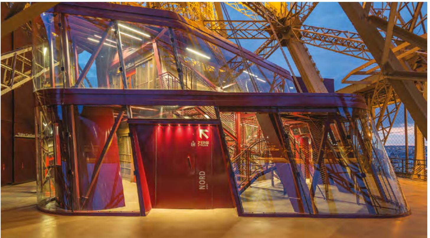
Fig. 9. Pagoda's glass façades for the elevators
