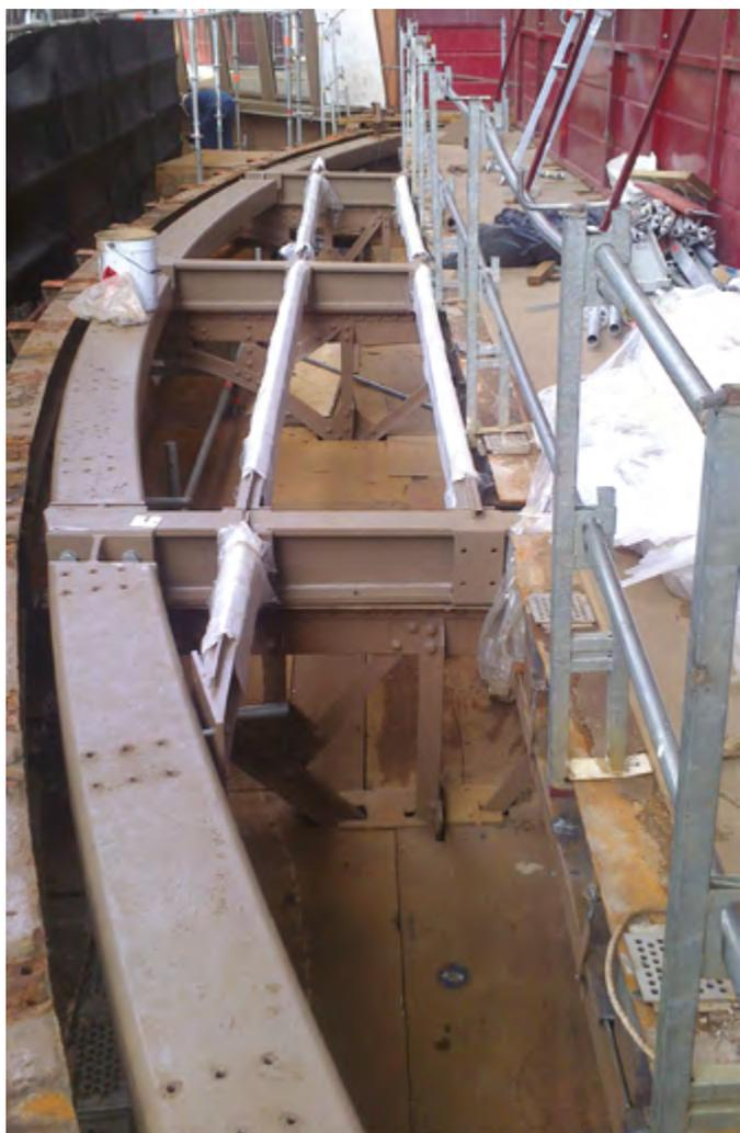
Fig. 10. Glass floor structure fitted to the existing Eiffel Tower's structure
