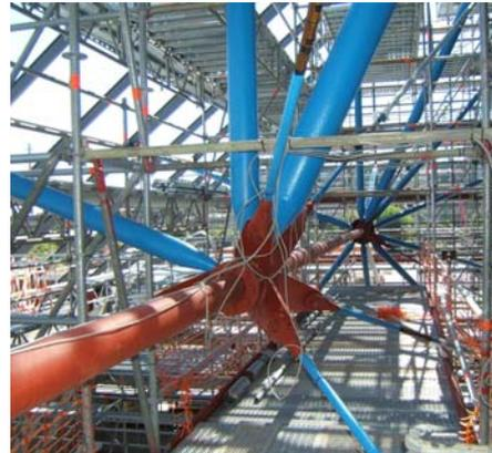
Fig. 5: The atrium just before being released from its connections to the scaffolding.
