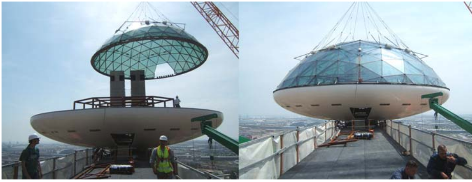
Fig. 5: Final positioning of the dome on top of the tower.
