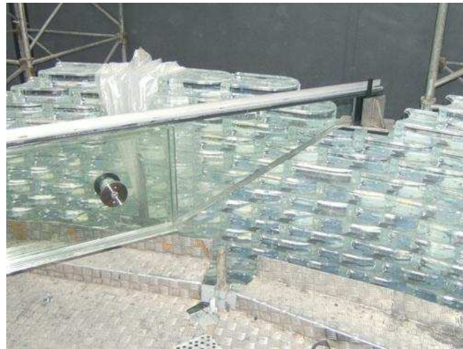
Fig. 9 - Glass girder on site
