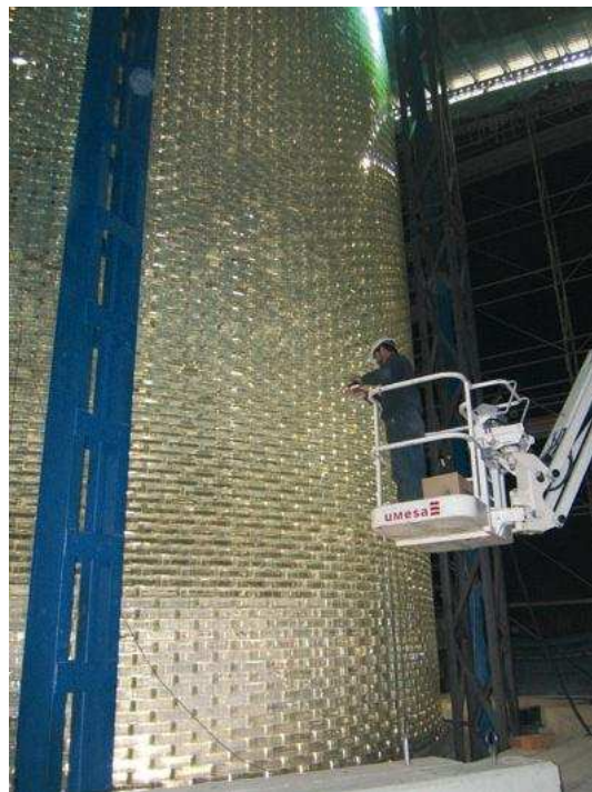
Fig. 7 - Sealing the glass wall
