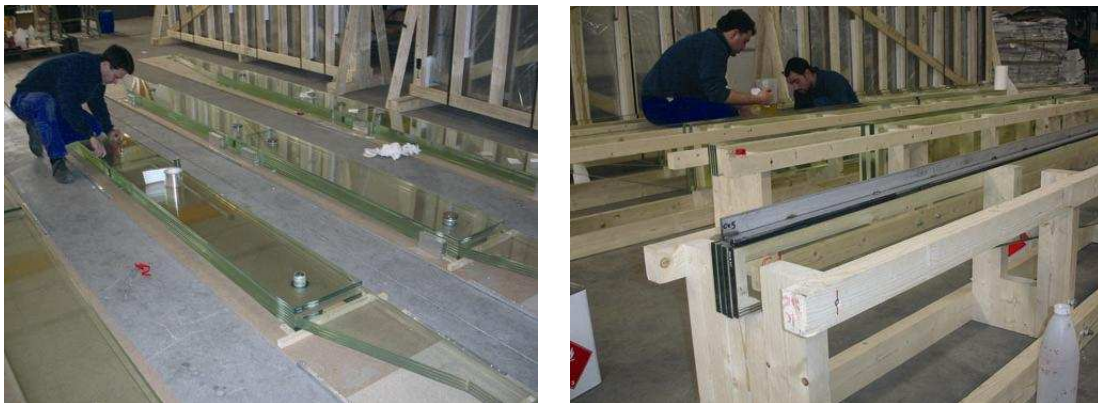
Fig. 8 - Fabrication of the glass girders
