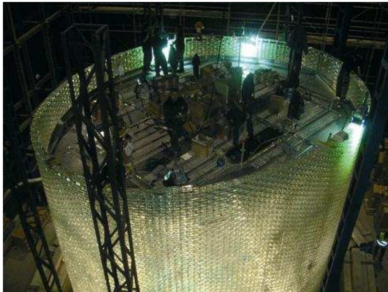
Fig. 6 - Glass wall during construction
