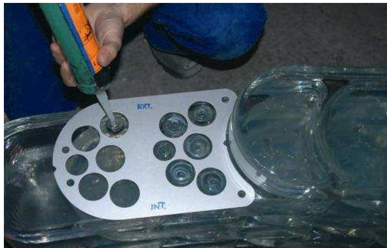
Fig. 5 - Distribution of adhesive on the glass blocks
